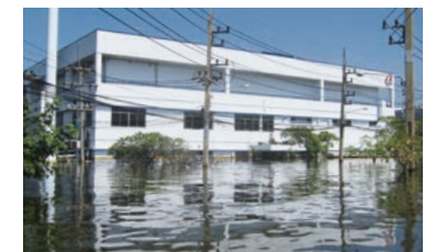
Medical factory inundated with 3 meters of water
