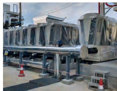
Replacement with high-performance chillers (Thailand Factory)
