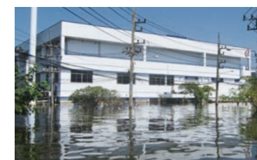
Medical factory inundated with 3 meters of water
