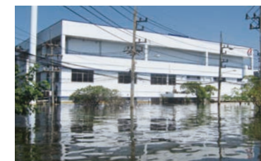
Medical factory inundated with 3 meters of water
