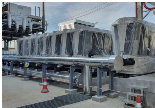
Installing energy-saving chillers
