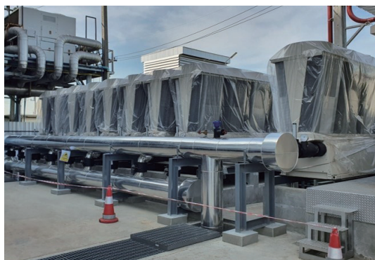
Installing energy-saving chillers
